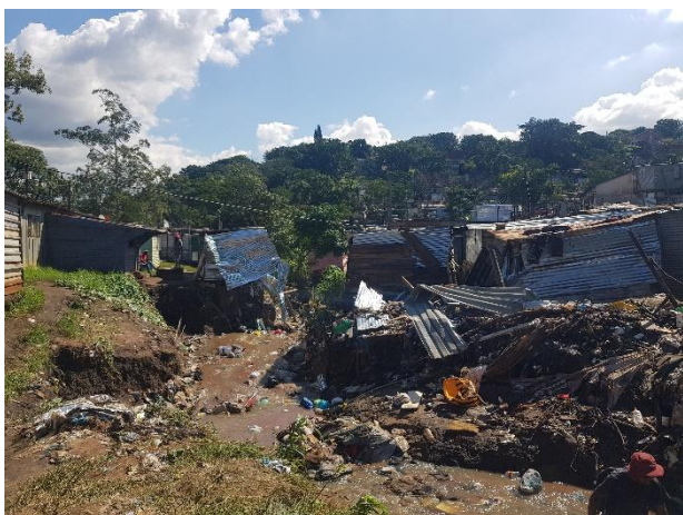
Figure 1 - Flood damage at Foreman Road
